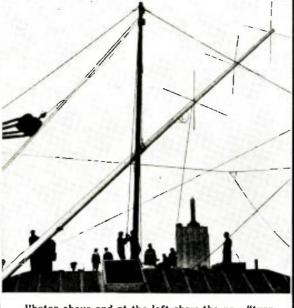
Photos above and at the left show the new "turnstile" antenna array in use at short-wave station, W8XH, Buffalo, N.Y. A 70 foot steel pole supports the antenna array; above—aerial being erected.
