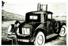
Fig. 5—400 mc. set in use as a "portable" on a car, with antenna arranged in a parabolic reflector.
